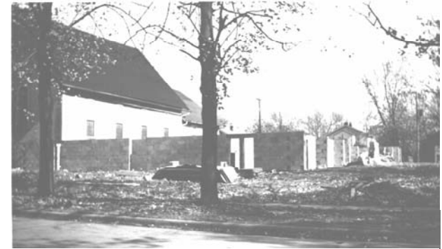
Looking east during construction in 1953.
